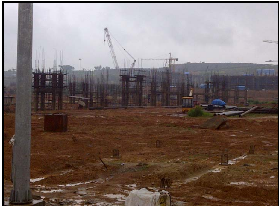
OMPL Mangalore Flare Site at the time beginning of Site Work
