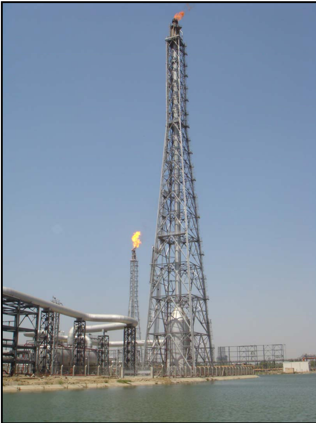
Flares in operation: 76" dia. X 130m Polymer+MEG Flare in front side AND 72" dia. x 119m NCU HC + Sour Flares in back side at IOCL Panipat Refinery, PNCP (EPCC-9)
