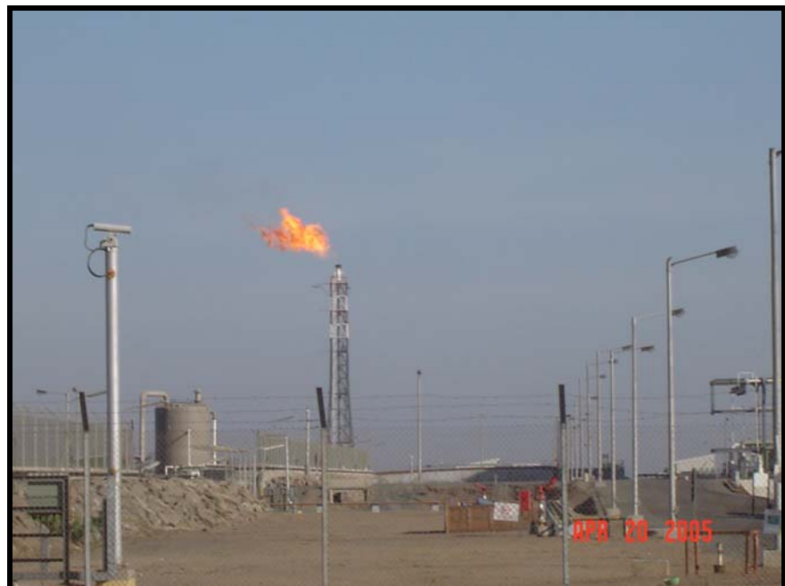
Flare (24" dia. x 52m high) in operation at Hazira Port & LNG Terminal
