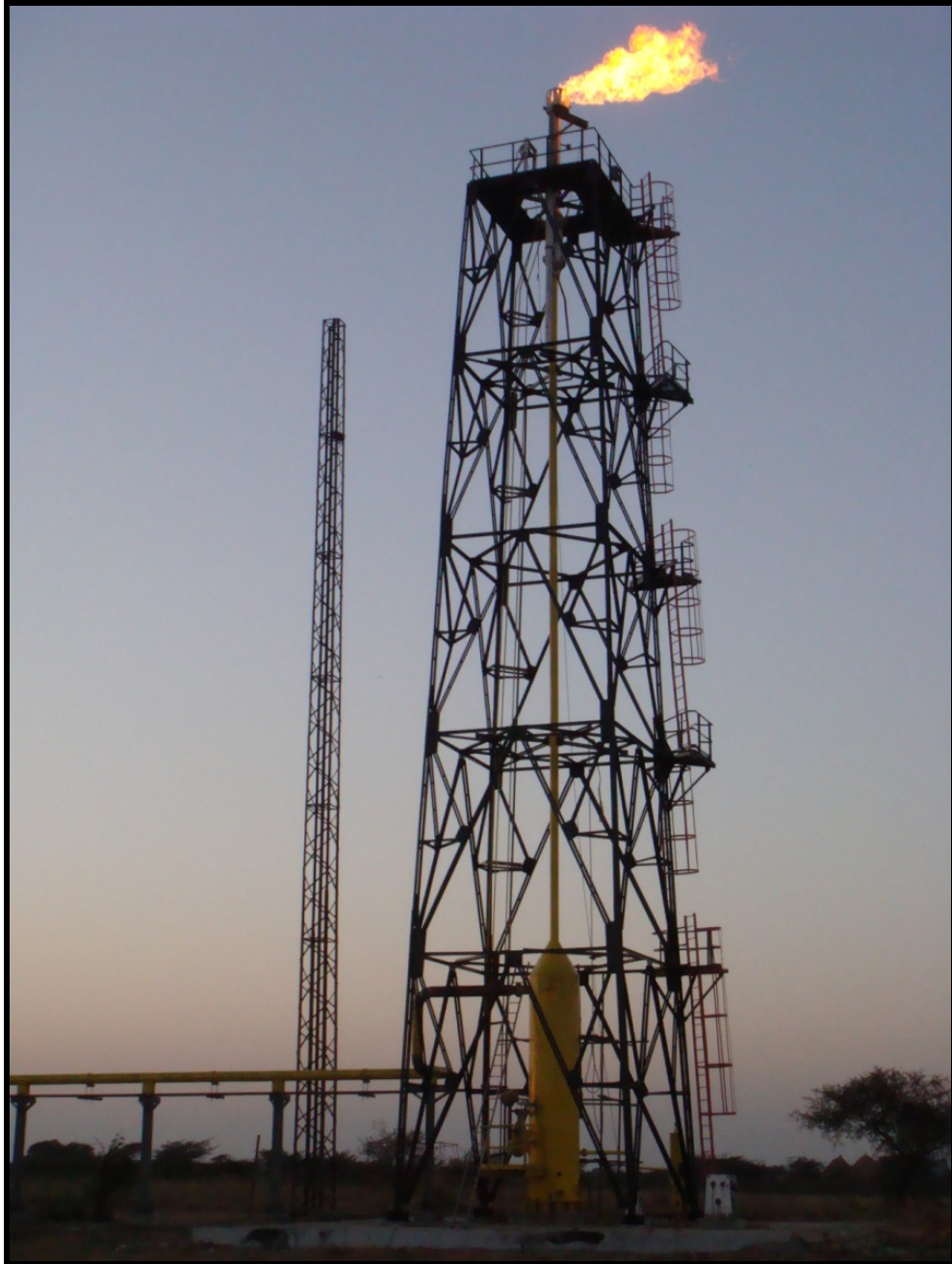
Flare (8" dia. x 30m high) for Expansion of GCS Olpad project of ONGC Ankleshwar, Gujarat
