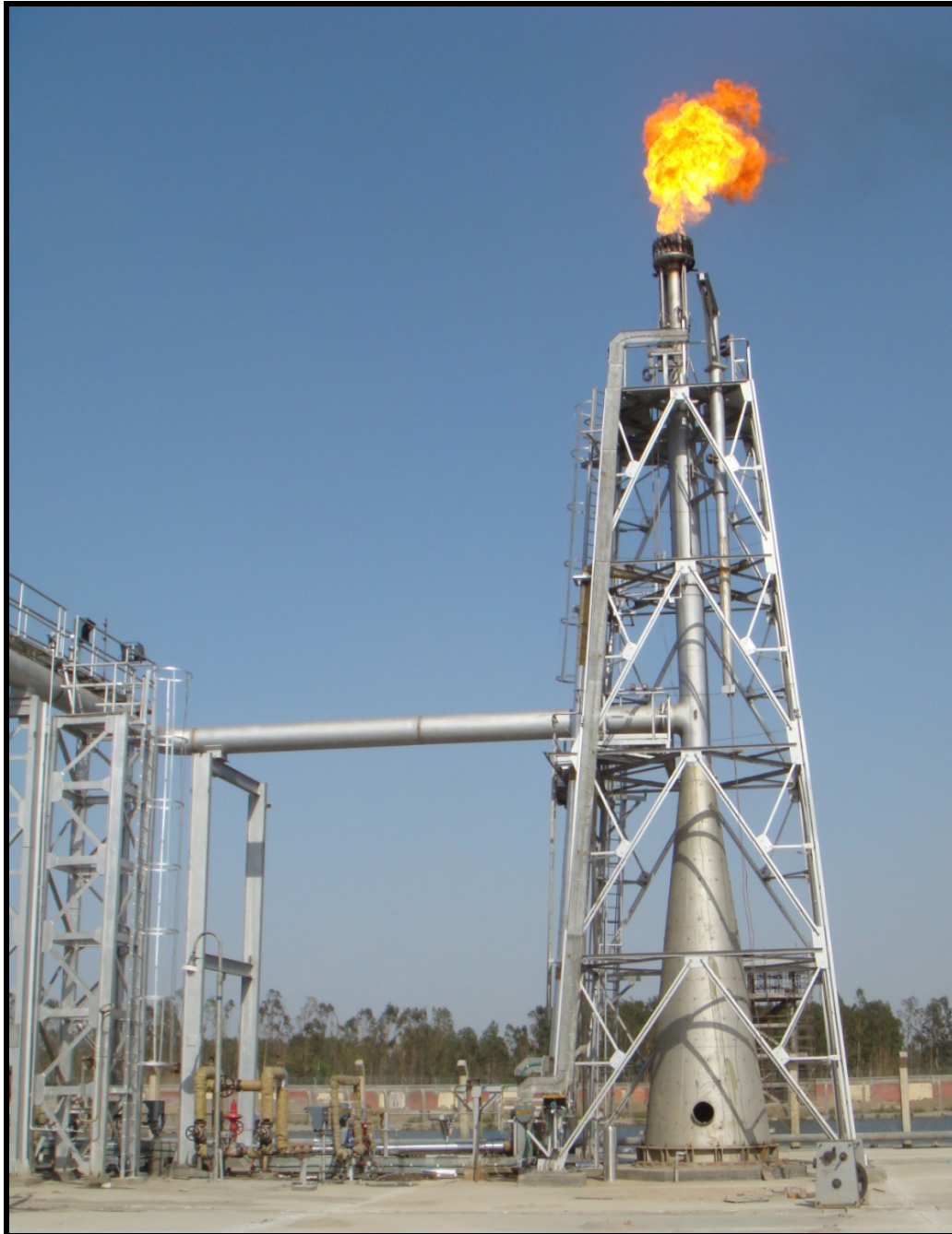
LP HC Flare (24" dia. x 20m high) at IOCL Panipat Refinery, Panipat Naphtha Cracker Project (EPCC-9)
